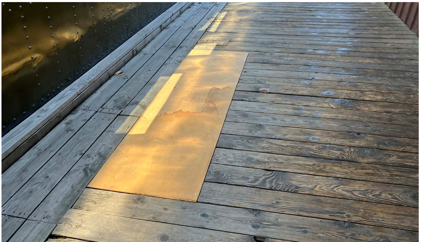
One of many patches that have been made over time
