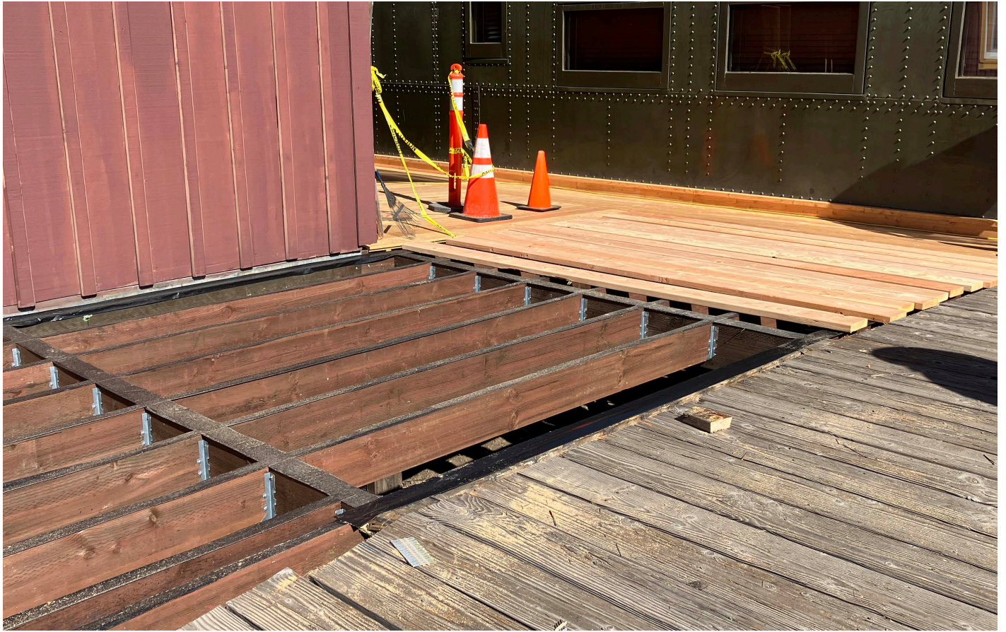
New structural pieces along the boardroom end of the Depot
