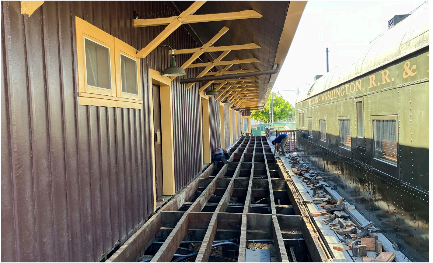
The planks along the track side of the Depot have been removed
