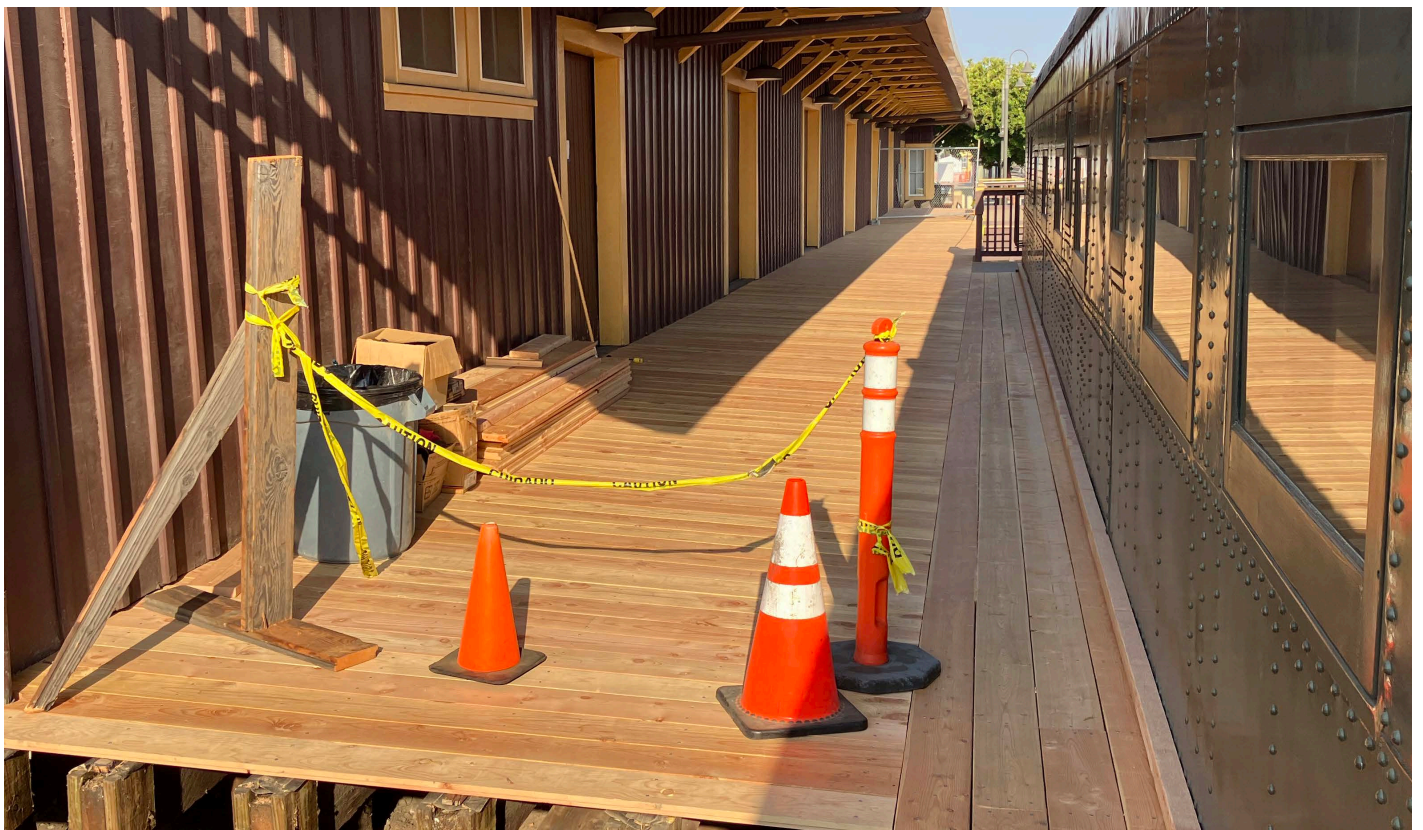
Boards between the deck and the railcar were also replaced
