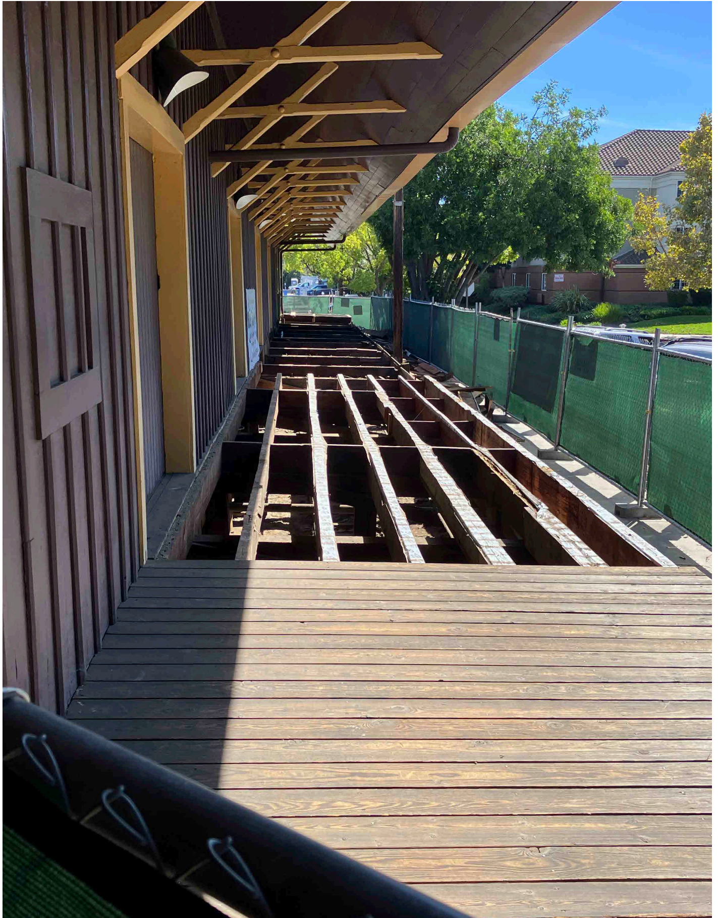
Just past the Depot entrance extensive repairs were needed to the supporting structure
